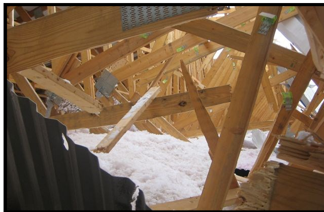
Interior photo of broken trusses of a collapsed hog barn
