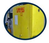
Are flammable liquids, fuel and oil kept away from any heat source and stored and labeled within an approved non-flammable cabinet?
