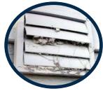
Dryers, within any confinement building or outbuilding, must have their exhaust vented to the exterior of the building. Check regularly for lint buildup.
